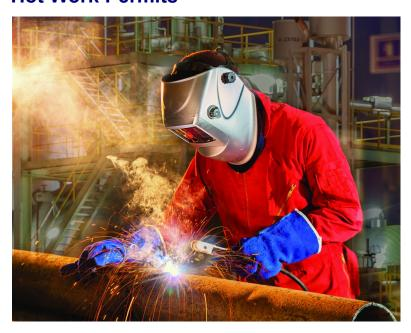
When performing any kind of hot work such as welding, cutting, or grinding, there are certain procedures to follow, required permits, and safe practices.
